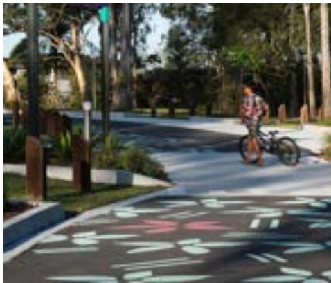
Safety for pedestrian by clear indication of shared roads
