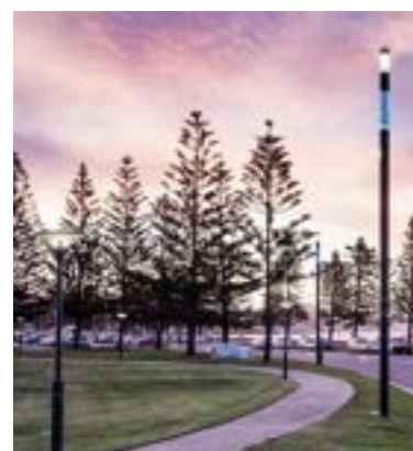
Dual street lighting for vehicles and pedestrians
