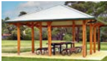
Upgrade of Shelter
