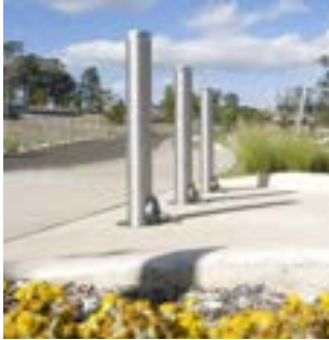
Removable bollards to allow site access along Foreshore Loop
