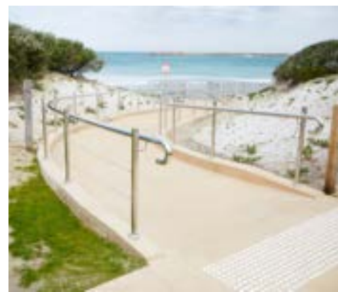
Accessible ramp to the beach
