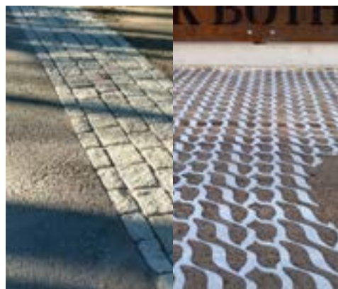
Rumble strip & Traffic calming measures
