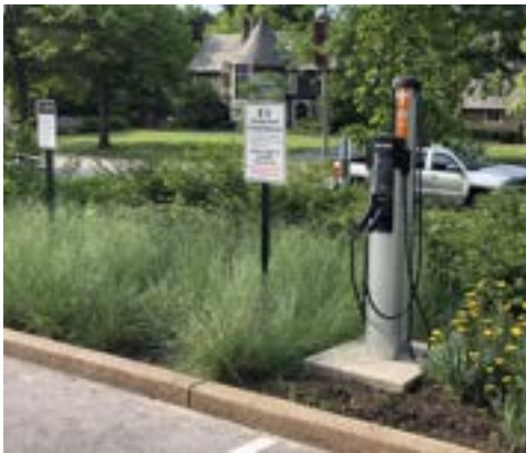
Dedicated EV parking
