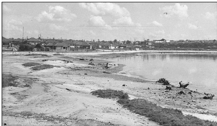
Figure 2.4: The final stages of reclamation of Iron Cove and creation of Timbrell Park – draining and filling behind the sandstone seawall at the head of the bay – in 1942 (Six Maps 2019)
