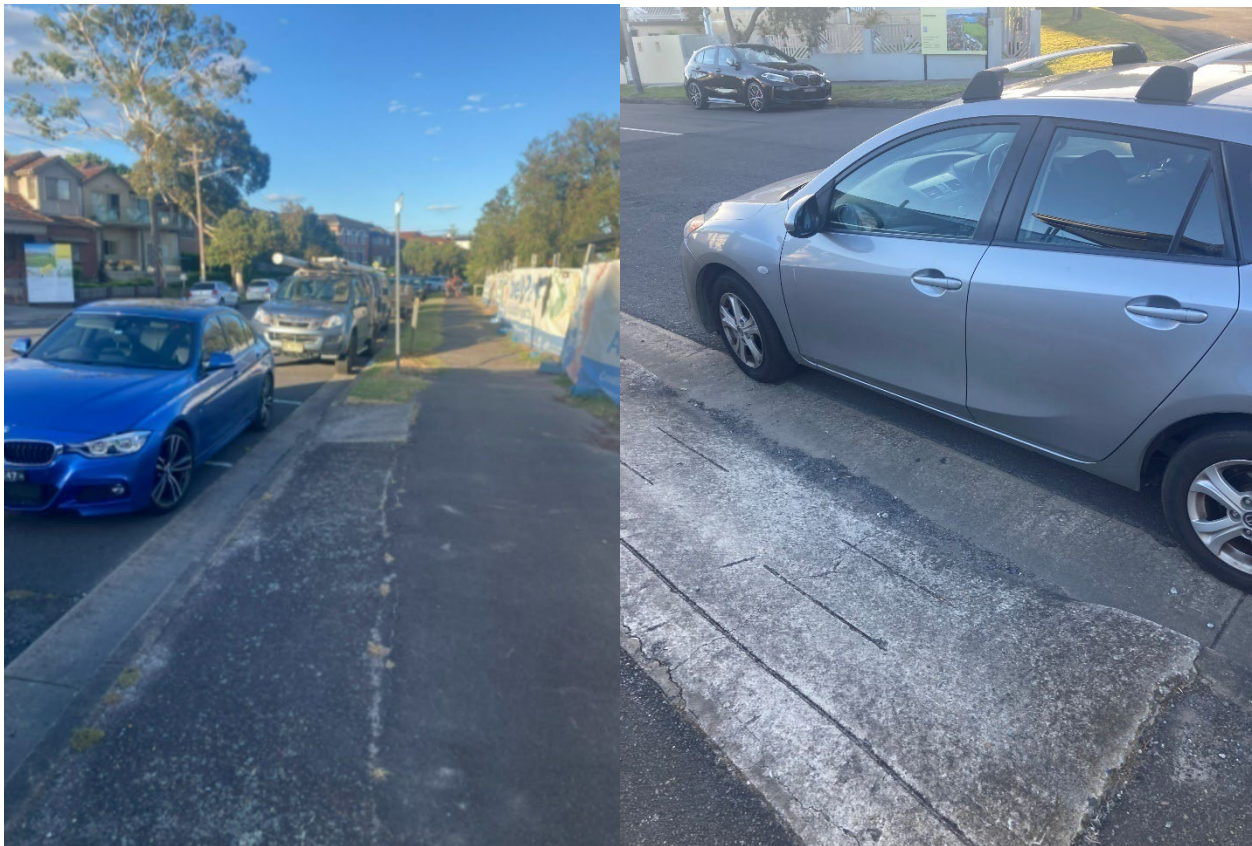
Figure 33 Parking Across Kerb Ramps
