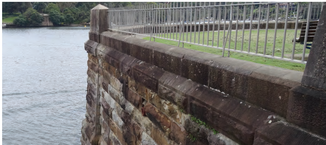
Western edge of abutment
