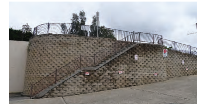
Marina stair access and driveway ramp
