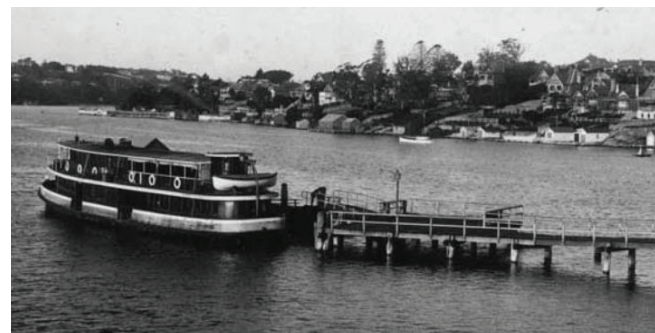
Old Gladesville Bridge ferry wharf
