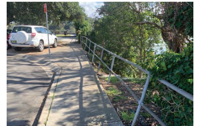
Vehicular damage to existing balustrade
