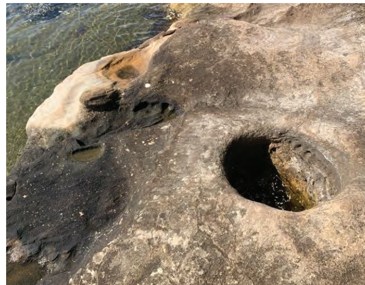
Old pier holes in existing sandstone shelves
