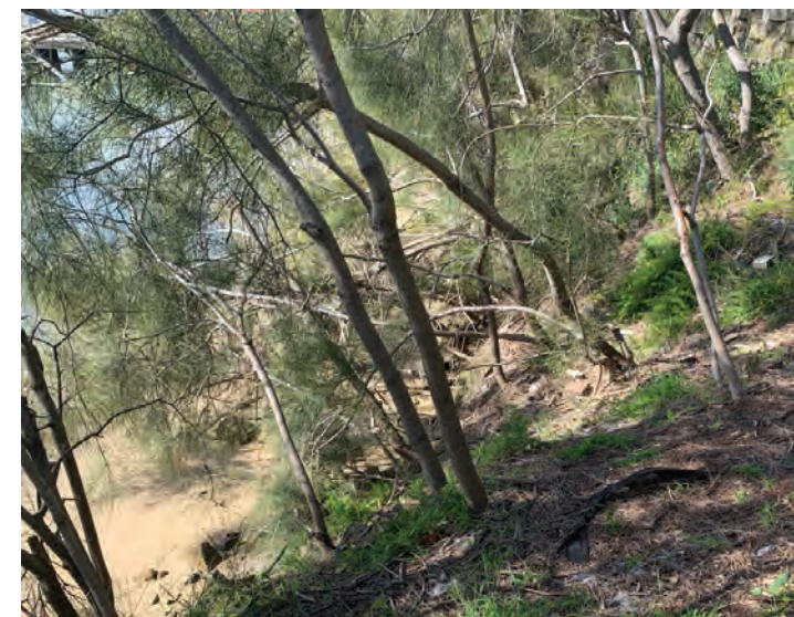
Self seeded Causaurinas along eroded eastern embankment
